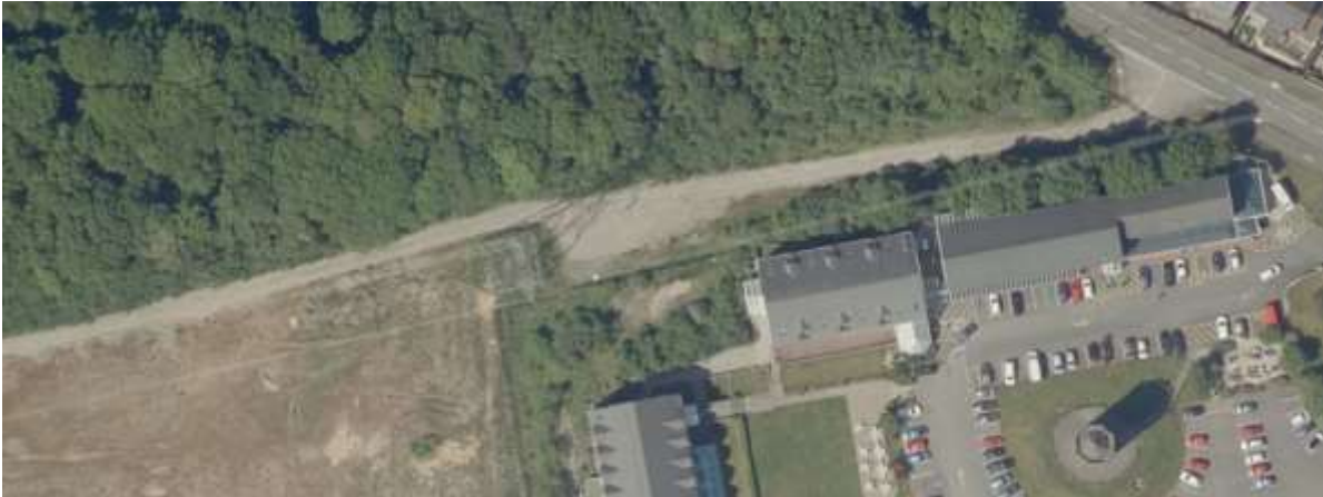
Figure 7: Existing Access to Site and Track
